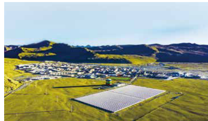
PV+Solar Thermal+Energy Storage Project, Tibet
